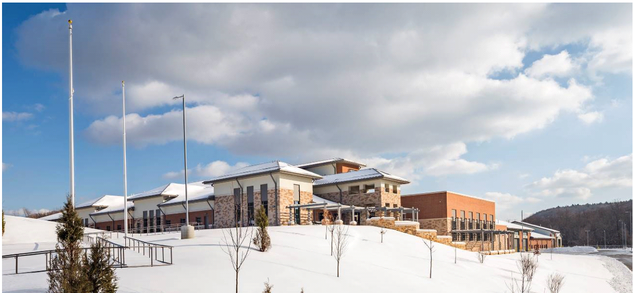
Project: Newtown Armed Forces Reserve Center at Danbury, Connecticut D/B RFP Preparer: RSP Architects Photo Credit: Korte-Fusco Joint Venture (D/B Contractor) / Michael Baker International (D/B DOR) © Robert Benson Photography
